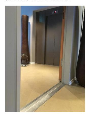
In front of the staircase and elevator area is a 3 cm high door steps with slope on each side. The door is 136 cm wide.
